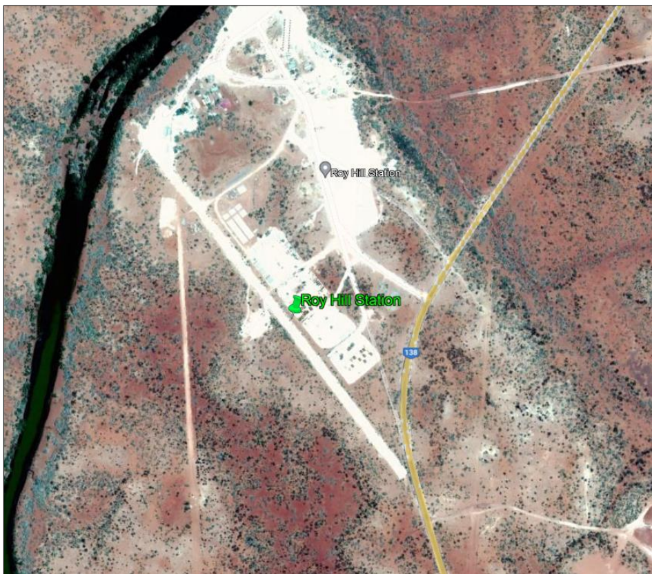
Figure 36: Roy Hill Station ALA 48
