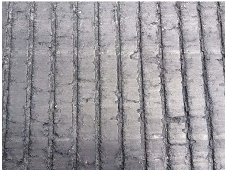
Figure 17. Example rubber contamination of a grooved runway.
