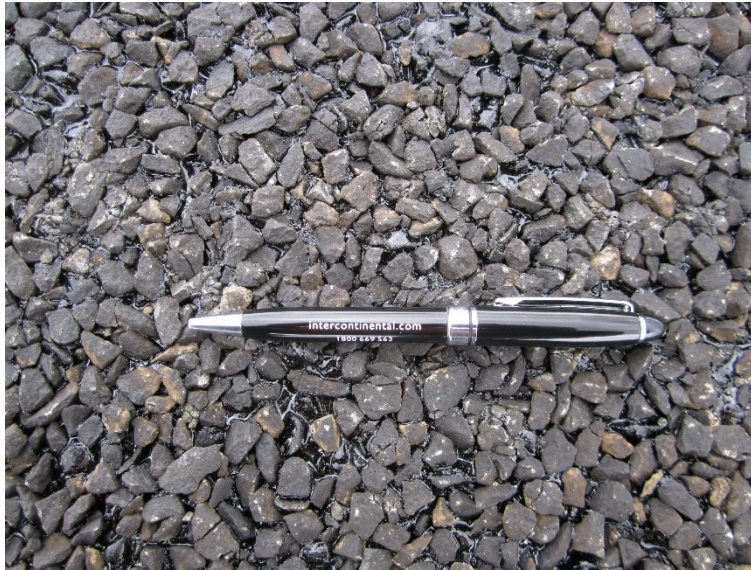
Figure 2. Typical sprayed seal runway surface.
