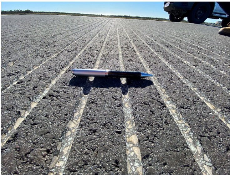
Figure 11. Typical trapezoidal grooves in DGA surface.
